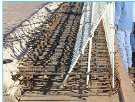
GFRP bars set up for barrier construction.
